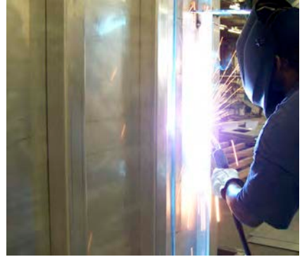
In-house or on-site welding
