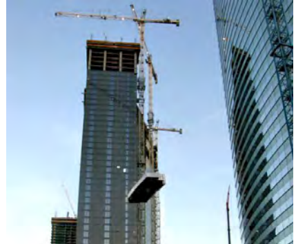
Craning whole vessel or large sections into place for elevated installations
