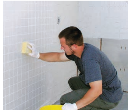
In-house or on-site tiling
